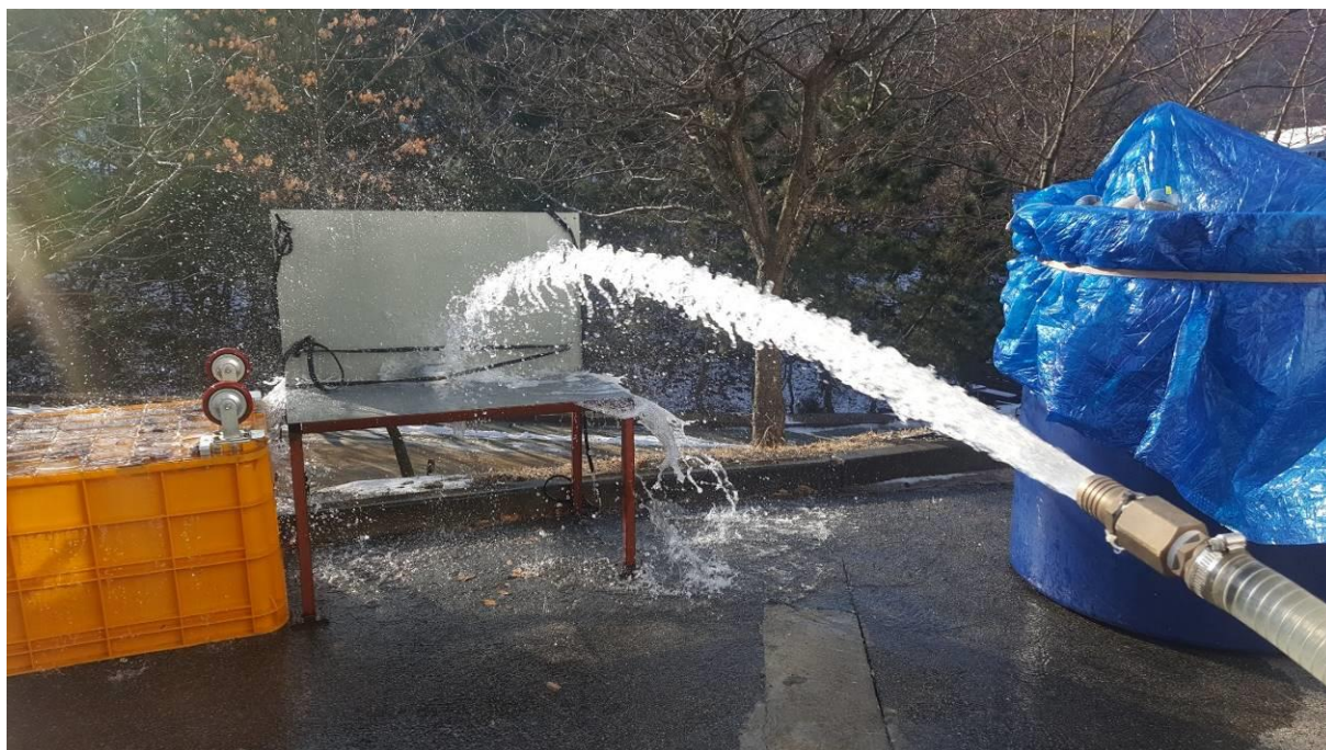
<Photo 3 > Hose down test
